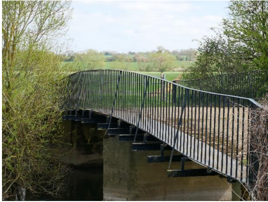
Sparsey Bridge over the Cherwell, adequate to take a cycleway
